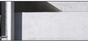
B. OFF FORM CONCRETE CANDALEPAS ASSOCIATES - ALL SAINTS PRIMARY SCHOOL
