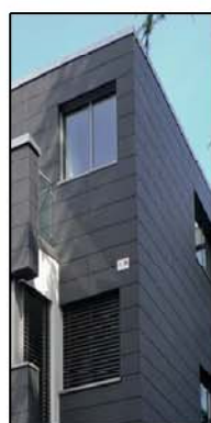
C. METAL CLADDING
